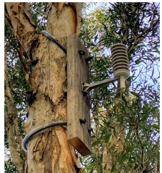
A tree-mounting solution that uses a hangboard. Straps are loose to accommodate tree growth, and are covered with rubber tube to protect the tree. The board is heavy hardwood that will not move in the wind, and blends in visually with the tree.
