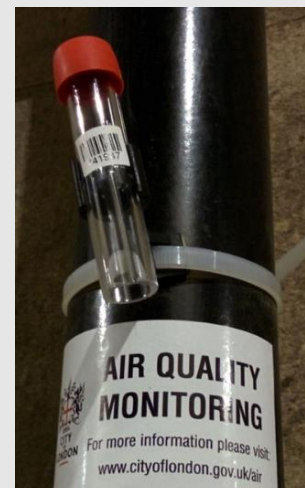
A gas diffusion tube used by the City of London. Image source: Creative Commons
