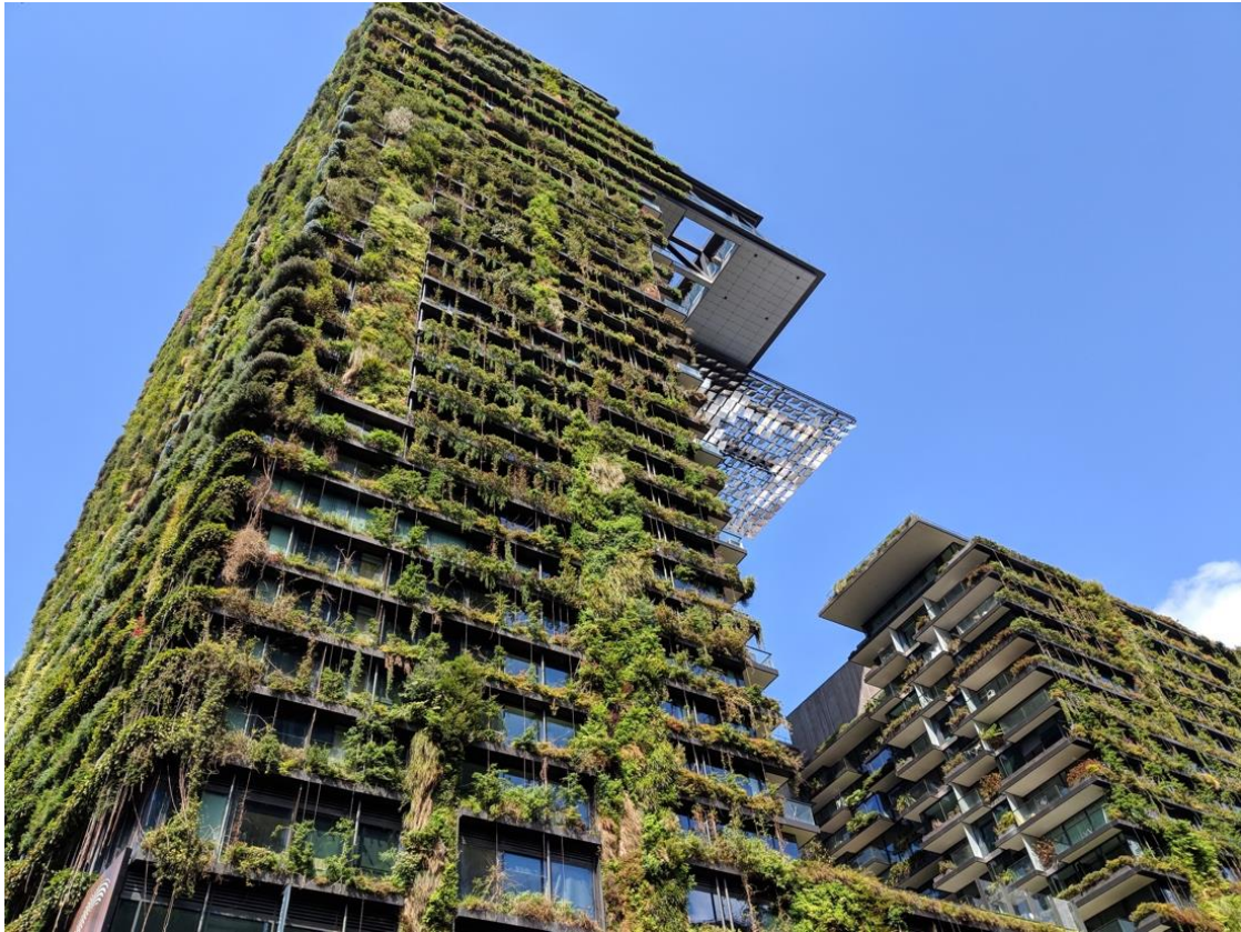
Green walls (like this one in Sydney, NSW) can actively clean pollutants from the air. Image source: Creative Commons
