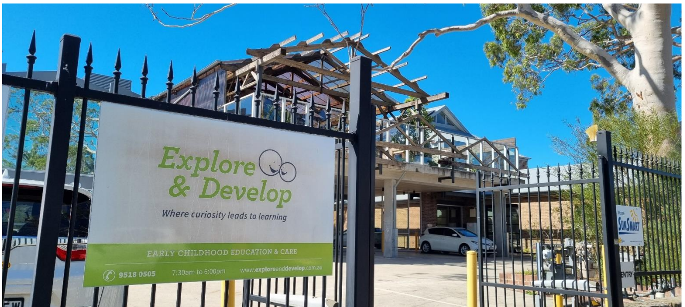
Vulnerable receptor sites (such as this childcare centre in Leichhardt, NSW) can be adversely impacted by air pollution. Image source: UTS
