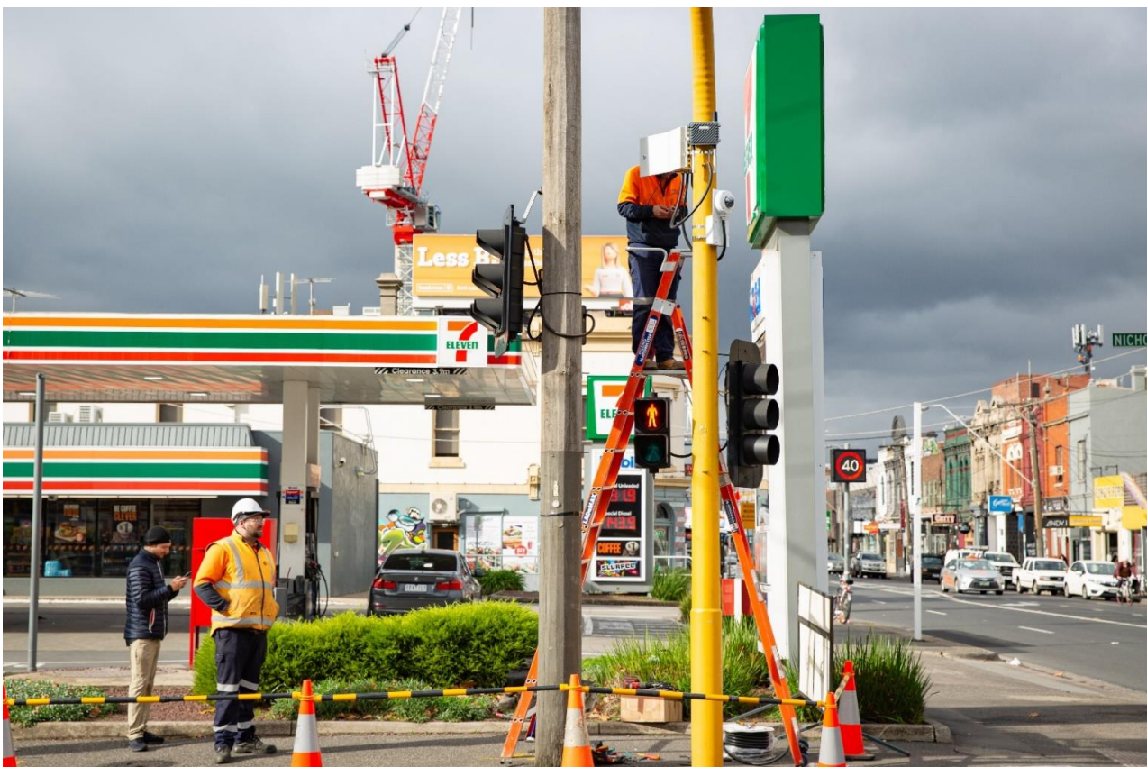
Smart traffic lights being installed in Fitzroy, Victoria. Image source: Cesar Nicolas, University of Melbourne
